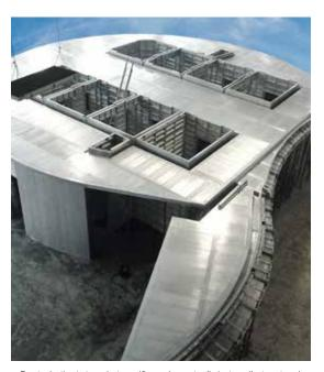
$\blacktriangle$  Exact adaption to to project specific requirements eliminates adjustment work on site and speeds up forming time
