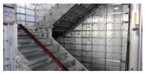
▲ Thanks to test assembly we can ervery time ensure the correct setup of the system - especially for special areas like as staircases, special shaped walls, etc.
