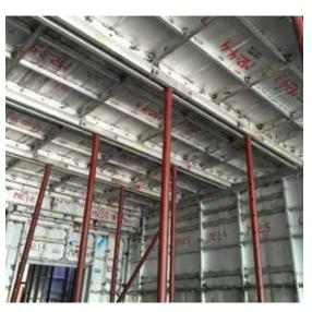
▲ Build smart - Doka Aluminum Formwork System produced by MFE allows highly cost-effective forming achieved by an adaptive and logical system concept
